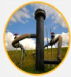
Wells are drilled at the landfill for landfill gas collection and are put under vacuum for central collection Biogas Clean Up
